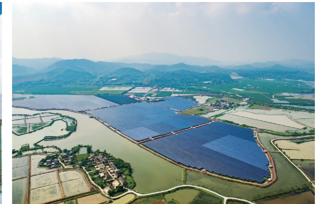
Fanchang Fishery-PV Complementary Solar Farm 繁昌漁光互補電站
