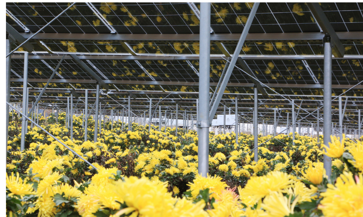
Planting golden chrysanthemums under solar panels in Xiaochang Solar Farm 孝昌電站太陽能板下種植金絲皇菊
