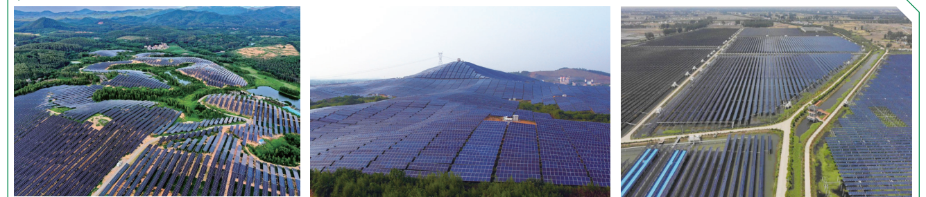
Heshan Agricultural-PV Complementary Project
